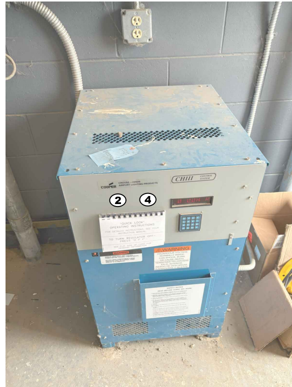
EXISTING L-828, 4kW CCR NOT TO SCALE
